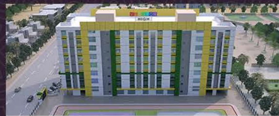
Vibgyor High School - Kharghar (0.3km)
